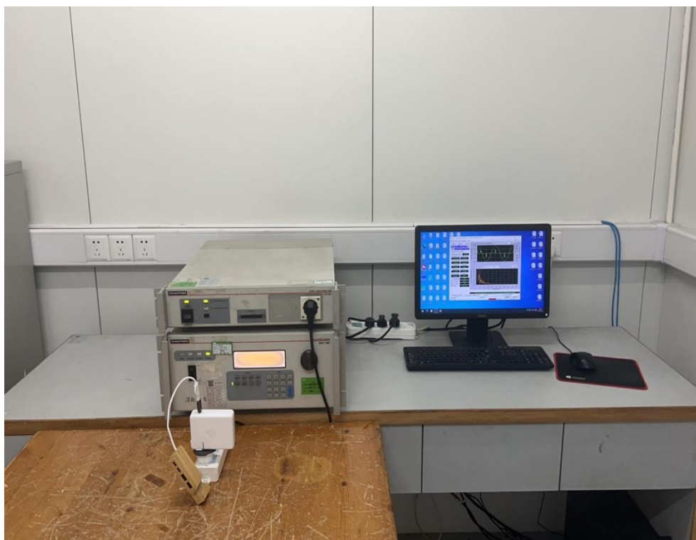
Harmonic current emissions & Voltage fluctuations and flicker
